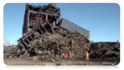
In 2016, the collapse of a boiler house at the Didcot Power Station in the UK resulted in multiple fatalities and injuries. While the exact cause of the collapse was investigated, deficiencies in maintenance procedures, communication between shifts, and inadequate documentation of structural integrity assessments were identified as contributing factors.
